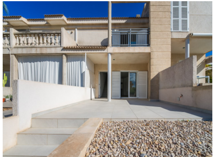
Terrace and exterior view
