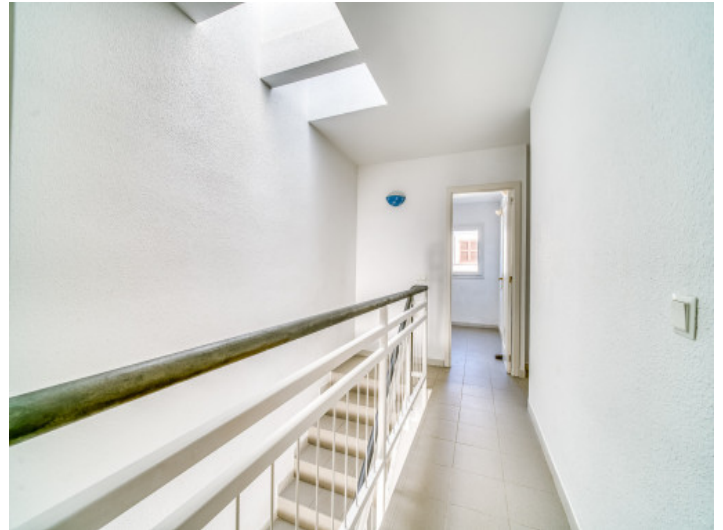
Corridor on the upper floor
